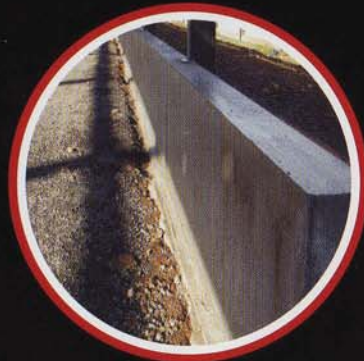
FINISHED SHUTTER WALL
