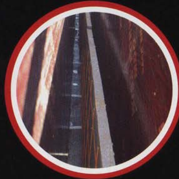
INSULATION AND REINFORCING INSIDE SHUTTER
